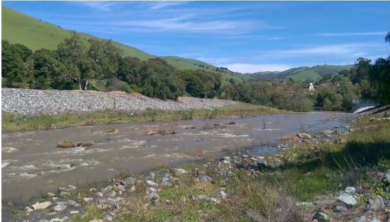
**Above:** Managed primarily for flood control and water management, this 12-mile reach to the Bay has engineered banks kept clear of vegetation. The bottom of the channel is flat, which leads to little diversity in flow and in-stream habitats.
